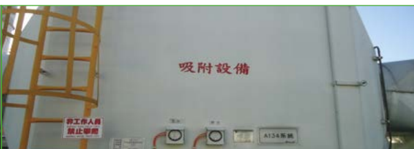
Activated Carbon Adsorption Tower
