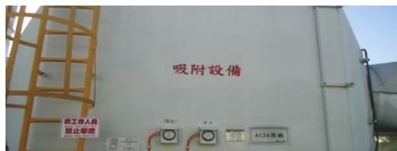
Activated Carbon Adsorption Tower
