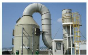
Air Pollution Control Equipment (Scrubber, Bag Filter, UVC Reaction Tower and Activated Carbon Adsorption Tower)
