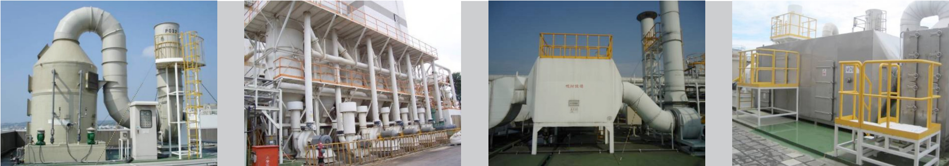
Figure 3.14 Air Pollution Control Equipment (Scrubber, Bag Filter, UVC Reaction Tower and Activated Carbon Adsorption Tower)
