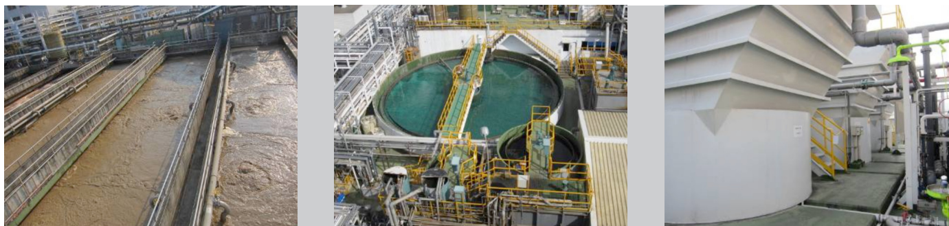
Figure 3.17 Photographs of Wastewater Treatment Equipment (biological ,coagulation and sedimentation ,and chemical reaction )
